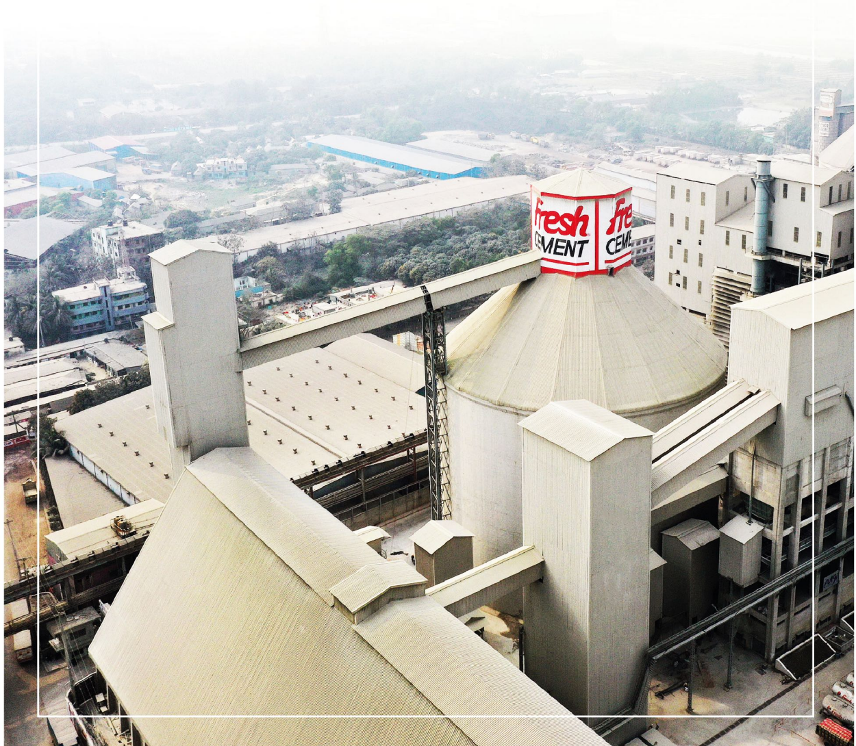
Aerial view of Unique Cement Industries Ltd. (UCIL)
