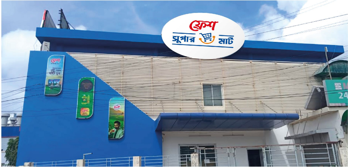
Newly renovated 'Fresh Super Mart'
